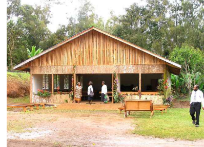
Our new church building still under construction. Price? $10,000
