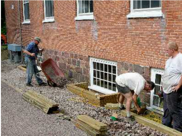
Church Member volunteers working. We have a completely new basement area.
